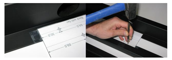
Drill the four holes. The result is shown on the right picture below.
